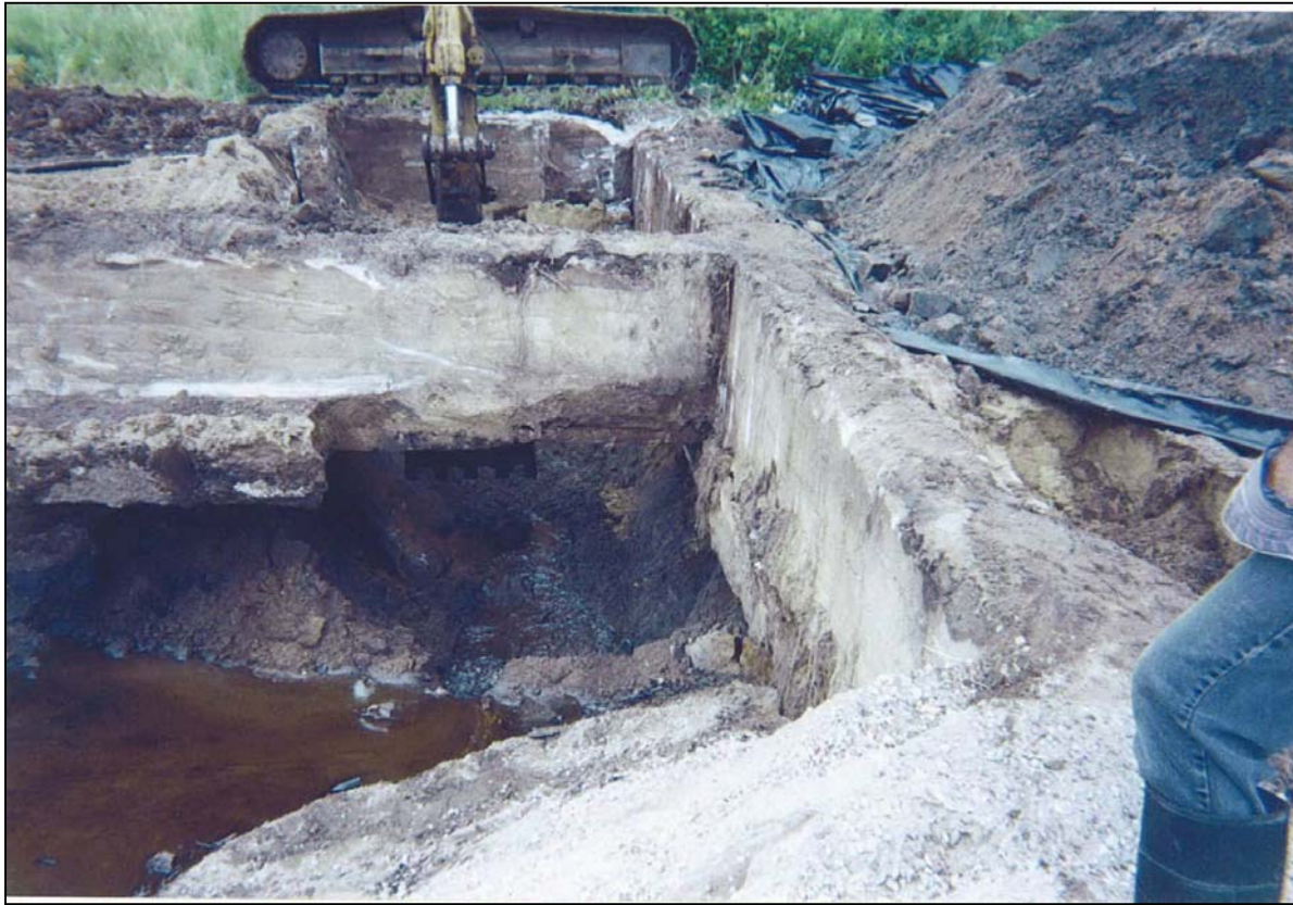
Figure 14 Foundations in the vicinity of the green material (Anson 00000027)
