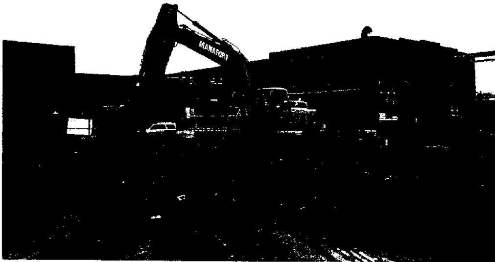
Photograph No. 2: Looking southeast from the north side of the former Building #16. Photograph shows the removal of the demolished concrete floor slab of former Building #16.
