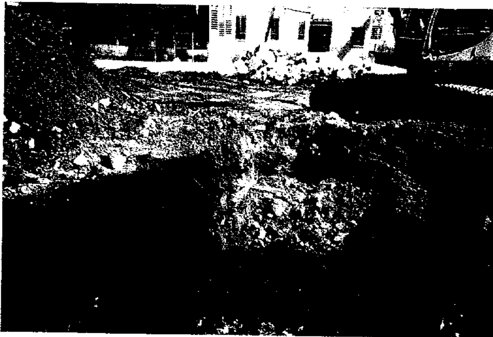
Photograph No. 10: Photograph of UST vault demolition. Fill material stockpile shown on the left side of photograph and concrete stockpile shown in the background.
