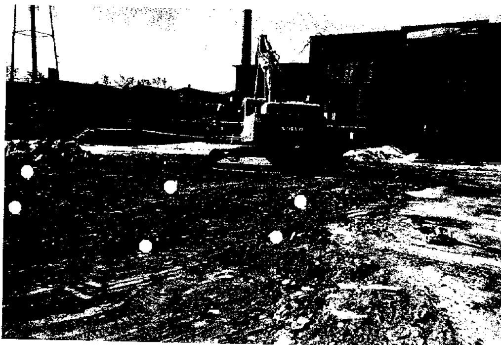
Photograph No. 3: Looking at northern portion of site. Some approximate locations for headspace volatile organic compounds (VOCs) screening indicated in yellow.
