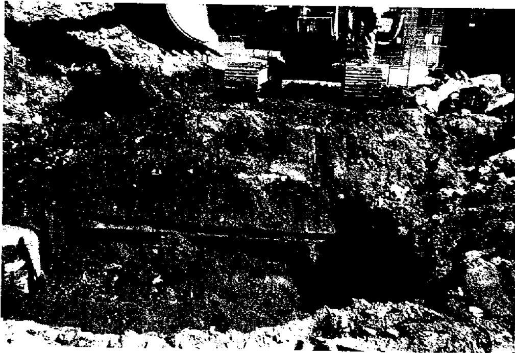
Photograph No. 6: View after southeastern vault wall removed. Two unknown pipes are identified, running north-south.
