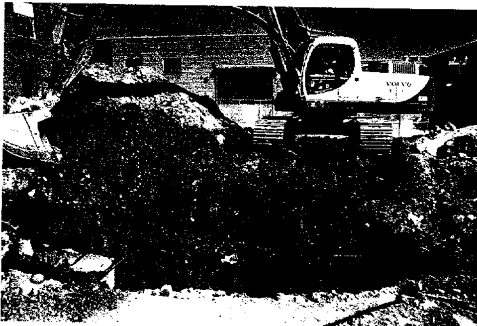
Photograph No. 7: Immediate backfilling required after southeastern vault wall removed to prevent rupture of two unidentified pipes due to weight of material stockpiled above.
