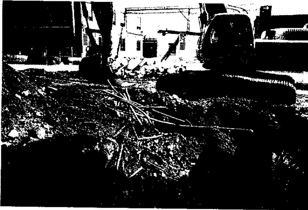
Photograph No. 1: Looking east at the exposure of piping leading towards UST vault area.
