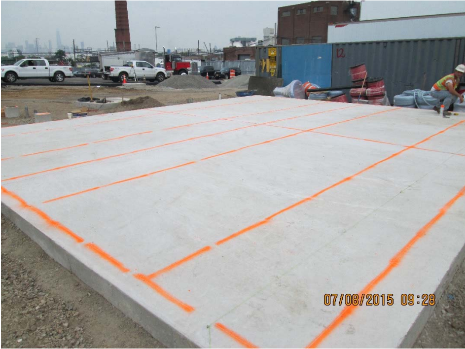
Photograph 7: Concrete pad for storage tanks
