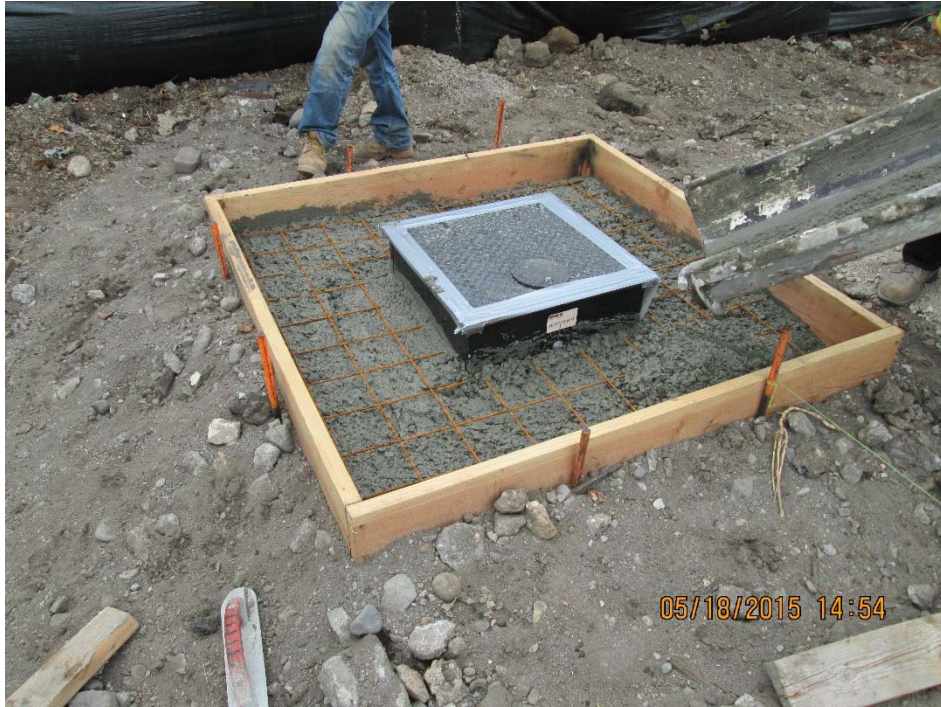
Photograph 3: Construction of well vault pad
