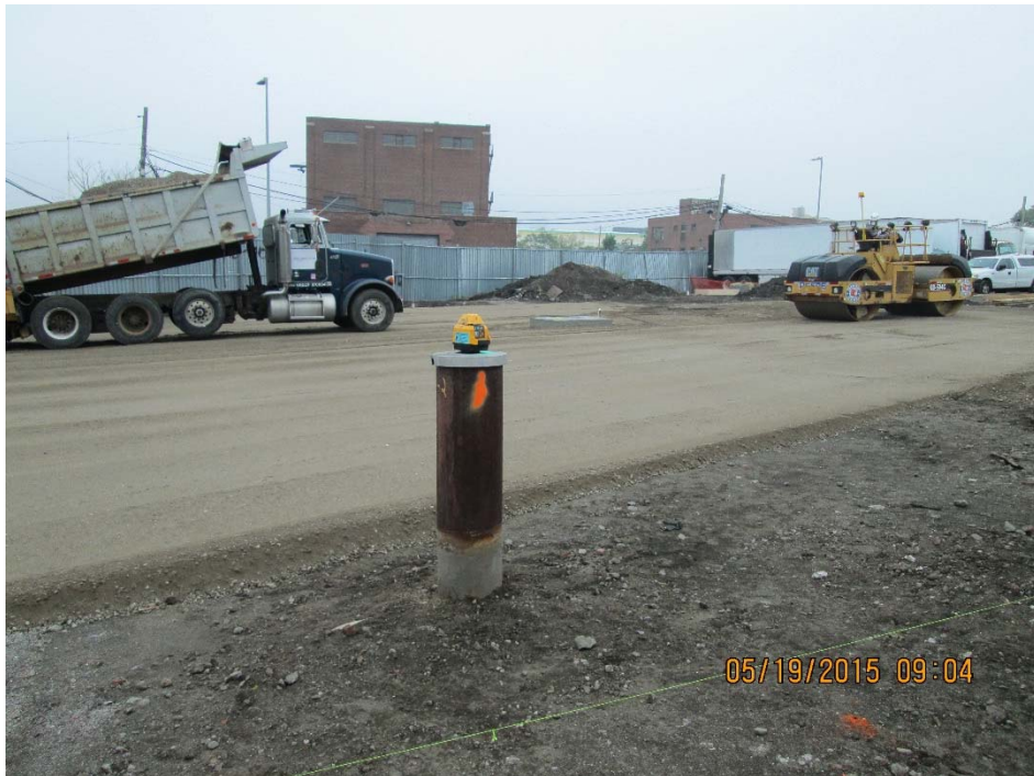
Photograph 4: Compacting DGA on RAD II
