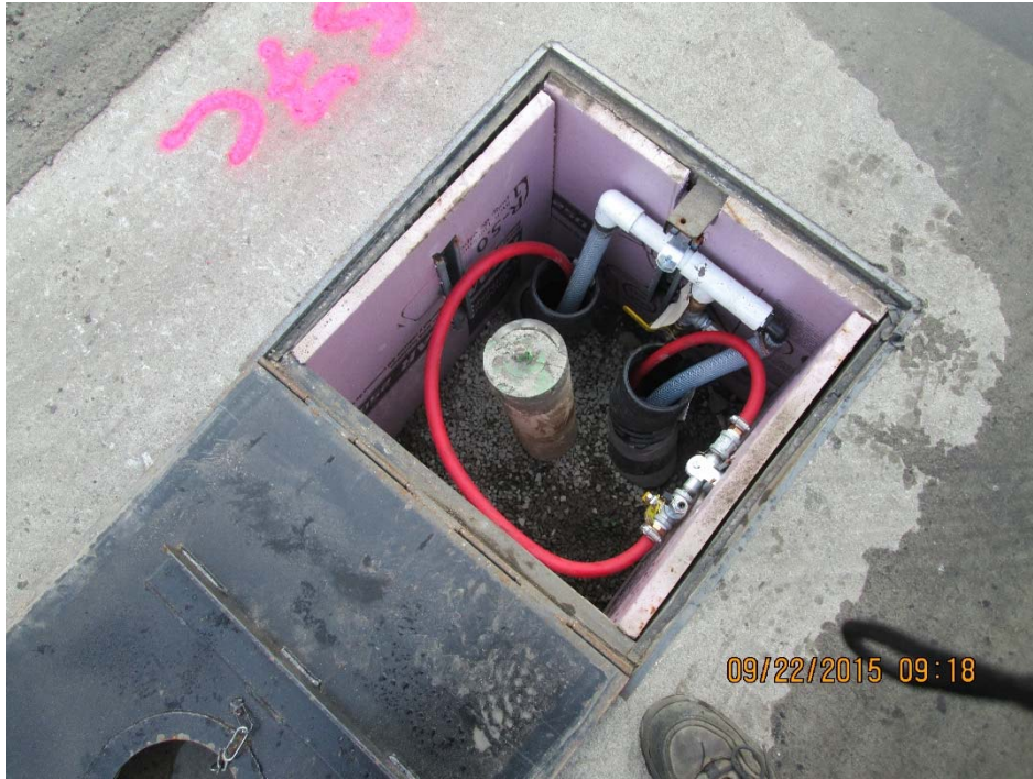
Photograph 15: Construction of recovery well piping
