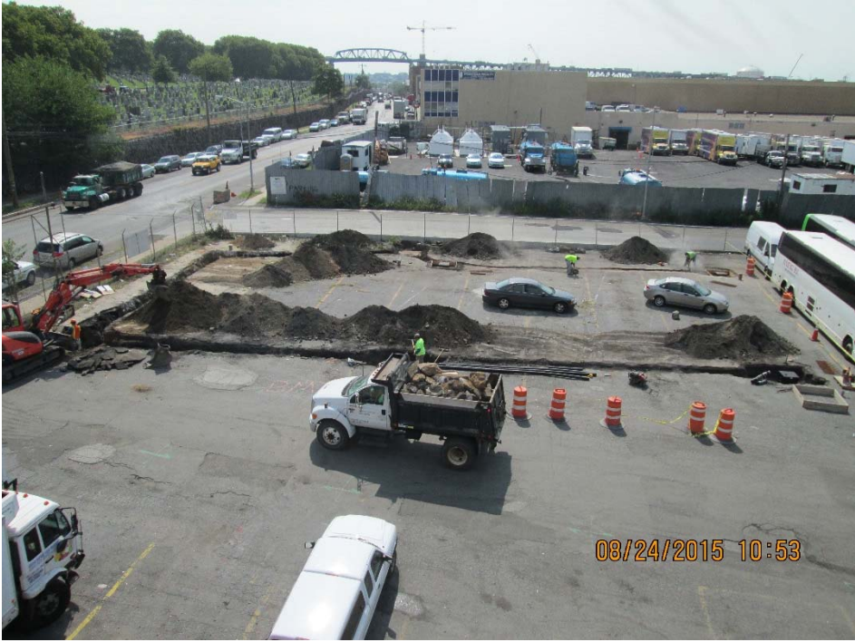
Photograph 11: Trenching operations on RAD I
