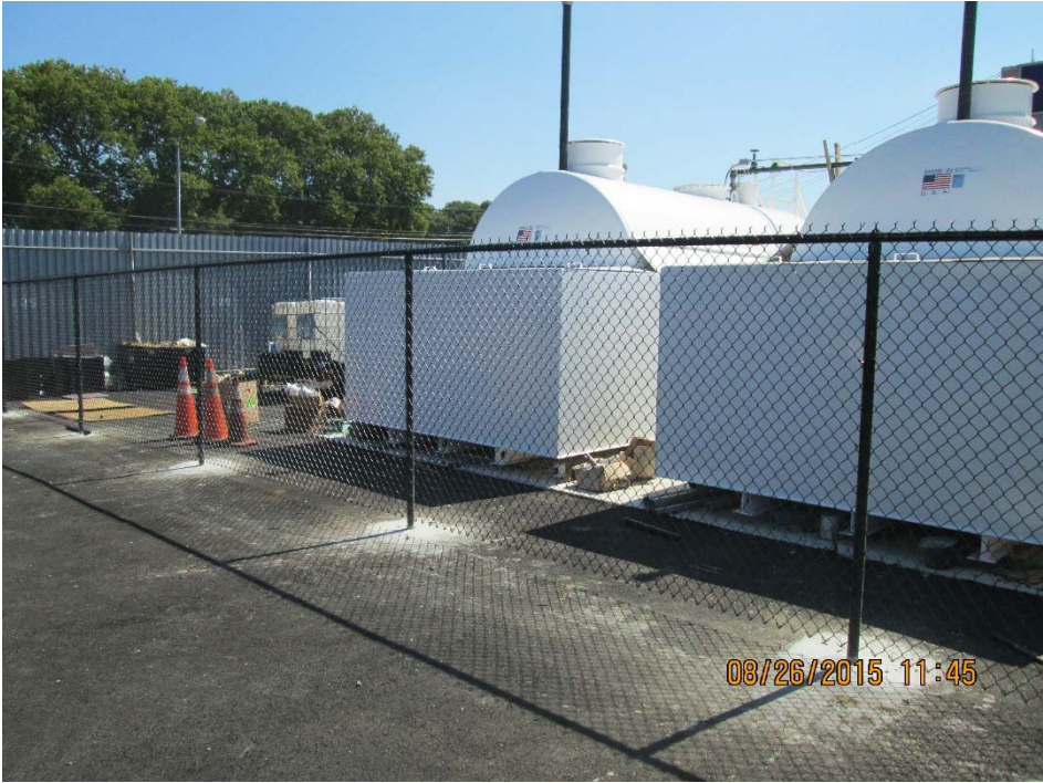
Photograph 10: Security fence around treatment area
