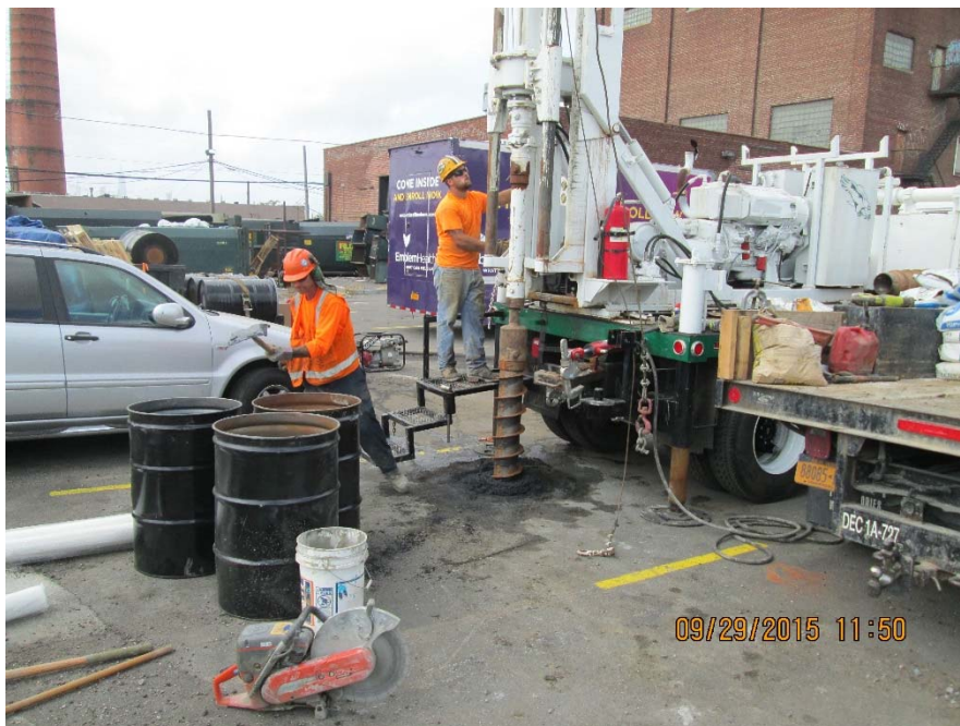
Photograph 16: Monitoring well installation
