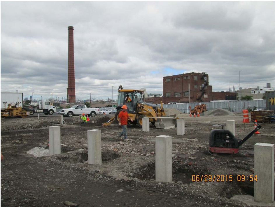
Photograph 6: Footings for equipment trailers
