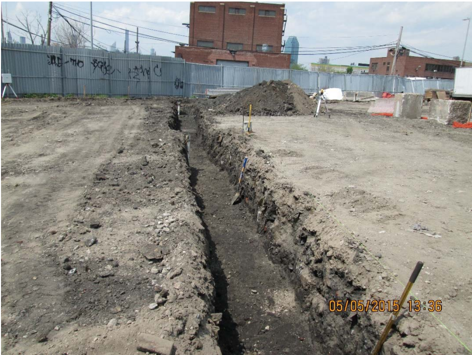
Photograph 1: TF-4 trench on RAD II
