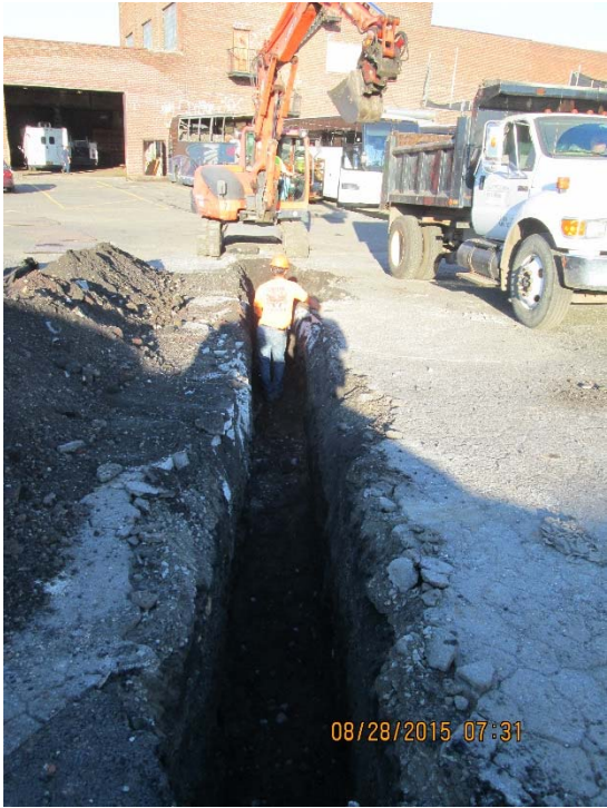
Photograph 12: Excavating trench on RAD I
