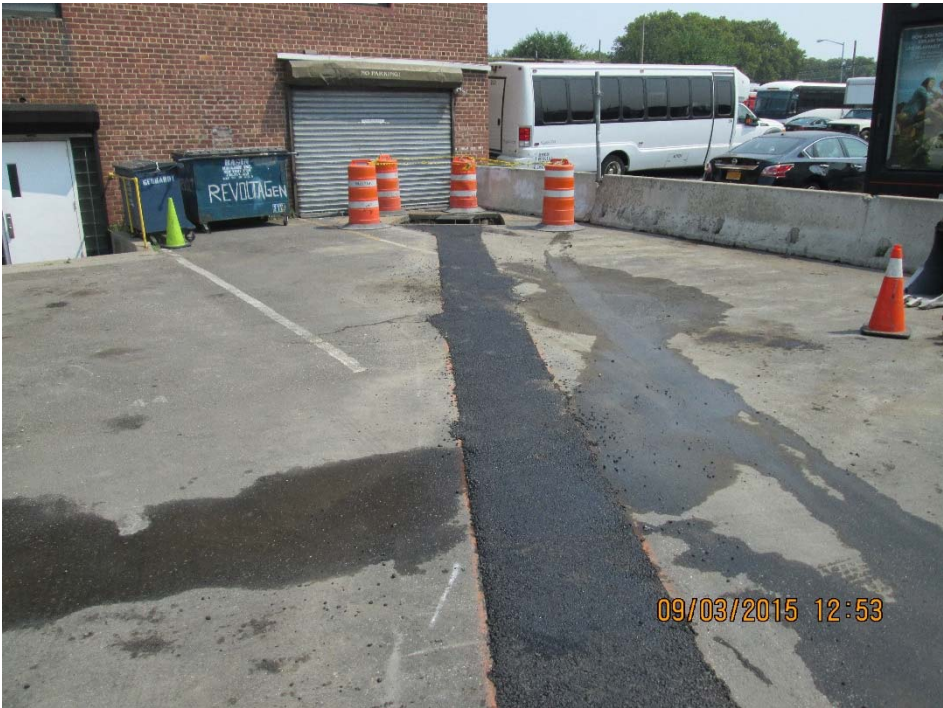
Photograph 13: Trench restoration on RAD I
