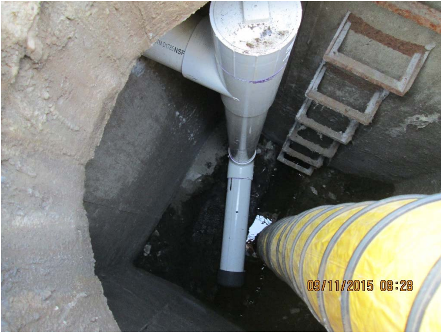
Photograph 14: Installation of force main sewer discharge pipe
