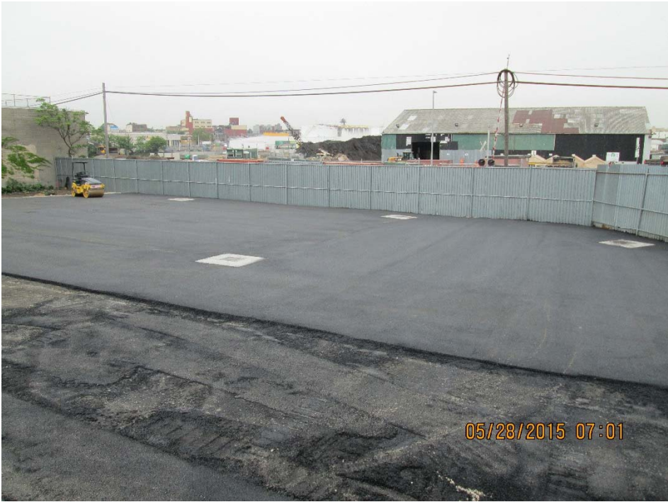
Photograph 5: New asphalt on RAD II
