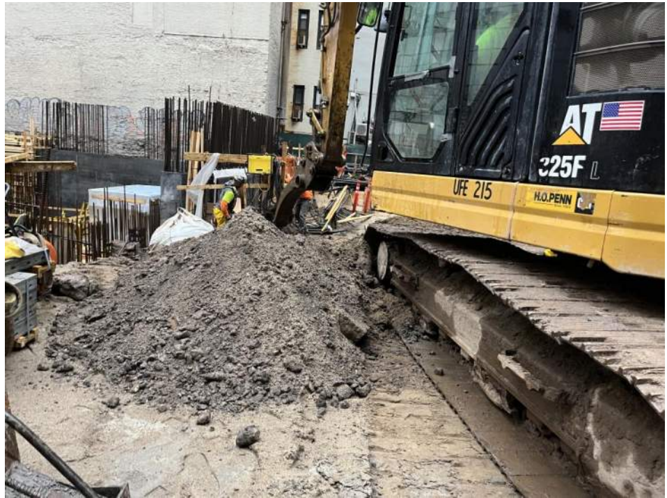
Photo 2: View of Urban excavating soil/fill in WC04 (facing northeast).
