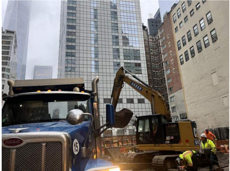
Photo 1: View of Urban loading a truck with soil/fill for export (facing northeast).
