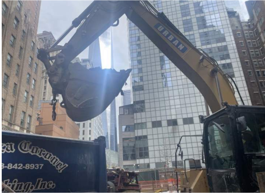
Photo 1: Urban loading a truck for soil/fill export (facing northwest).
