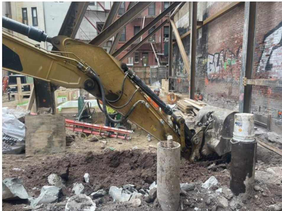
Photo 2: Urban excavating soil/fill in the southwestern area of WC04_0-5 (facing southeast).
