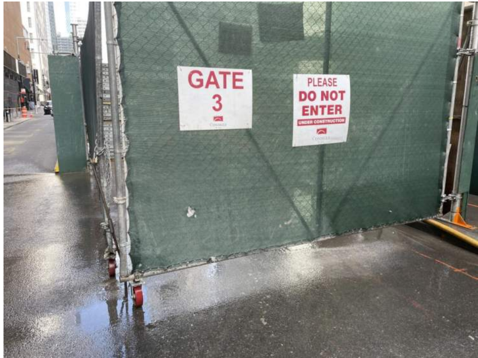
Photo 3: View of the site entrance/exit on Washington Street (facing northeast).
