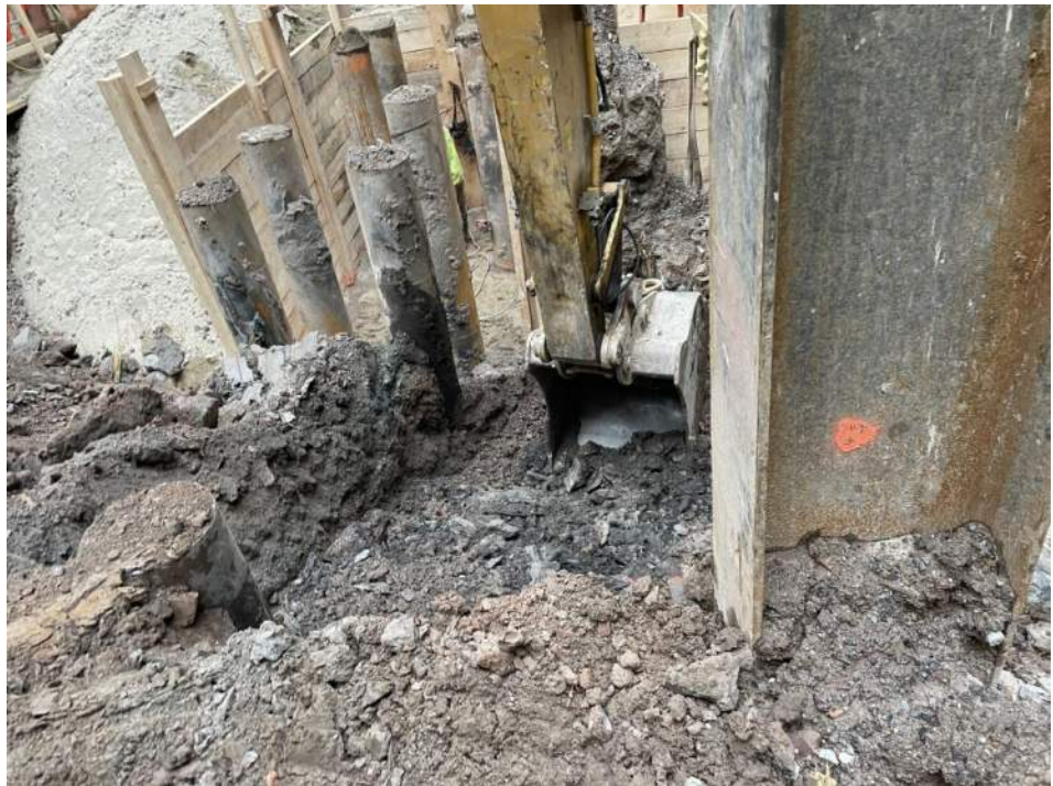
Photo 2: Urban excavating non-native soil with residual/ weathered petroleum impacts observed in grids WC05 (facing east).
