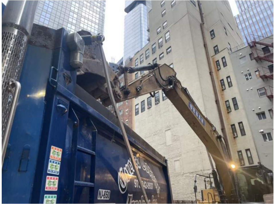
Photo 1: Urban loading a truck with soil/fill for off-site disposal (facing northeast).
