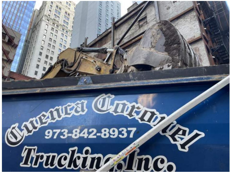
Photo 1: Urban loading a truck with soil/fill for off-site disposal (facing southeast).
