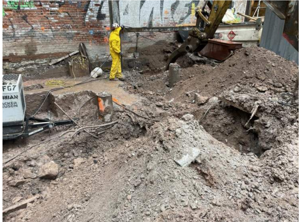
Photo 1: Urban excavating soil/fill in the southern part of WC05 (facing southwest).
