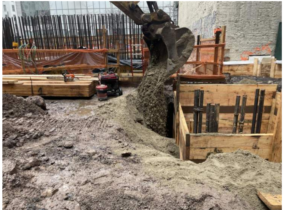
Photo 2: Urban backfilling in the eastern part of WC05 with imported pipe sand (facing north).
