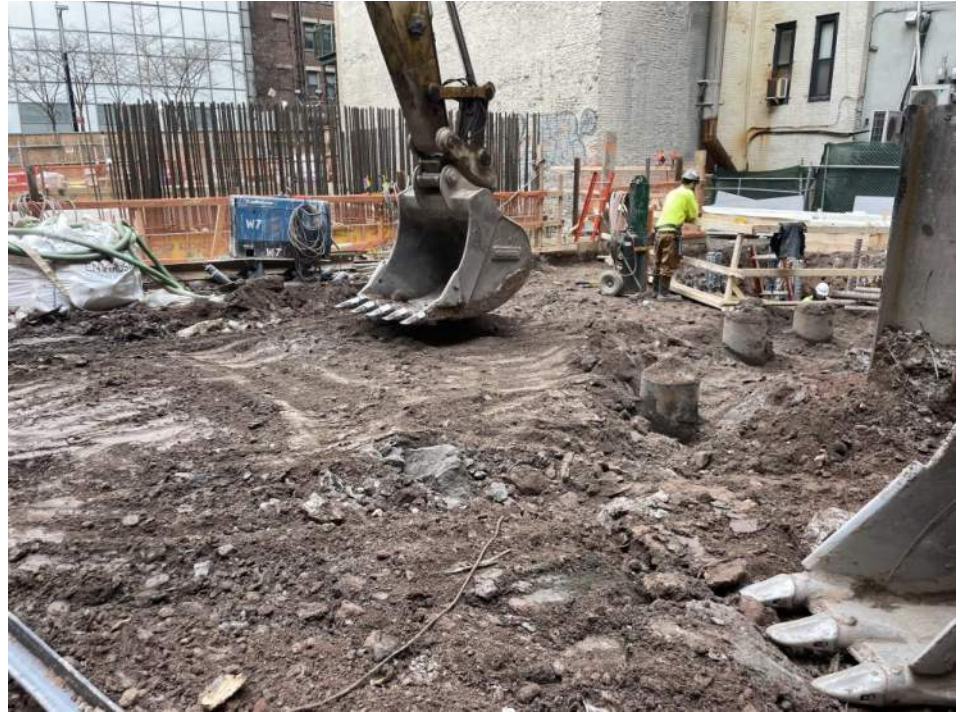
Photo 1: Urban grading soil/fill for equipment mobilization in grid WC05 (facing northeast).
