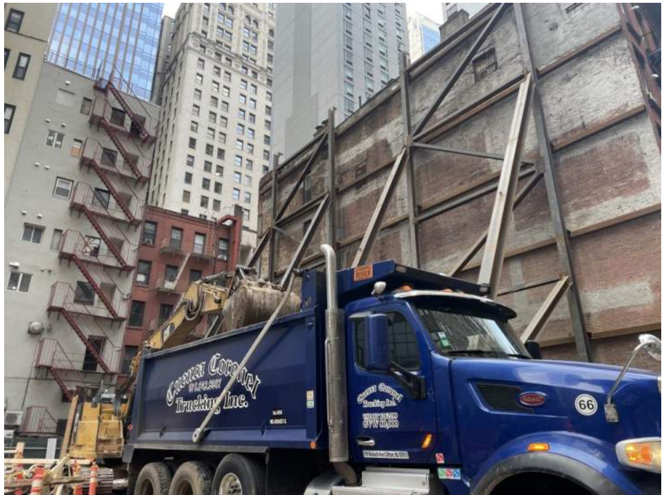
Photo 2: View of Urban loading truck for export (facing southeast).
