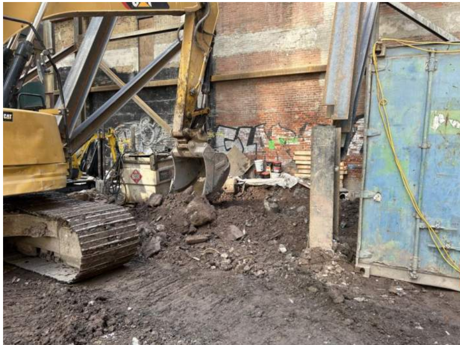
Photo 2: Urban excavating soil/fill in the southern part of WC04 (facing south).
