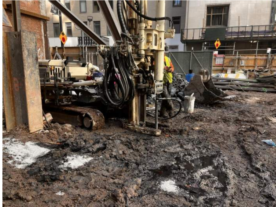
Photo 1: View of Brookside and Coastal injecting batch-mixed PetroFix® in the southern part of the site (facing northwest).
