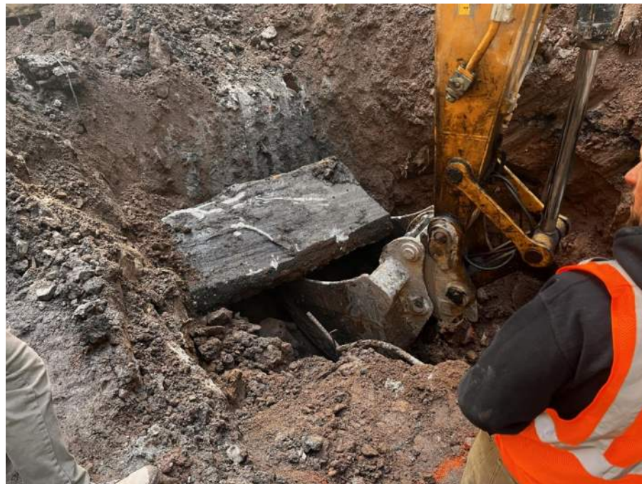
Photo 2: Urban removing concrete in grid WC04 (facing east).
