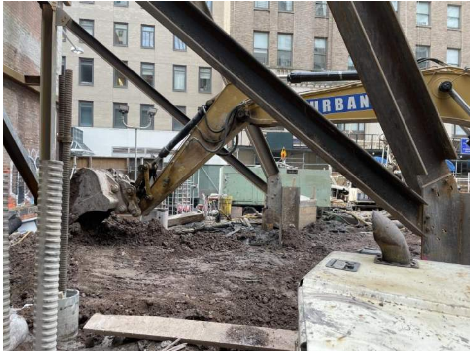
Photo 2: Urban grading soil/fill in grid WC04 (facing west).
