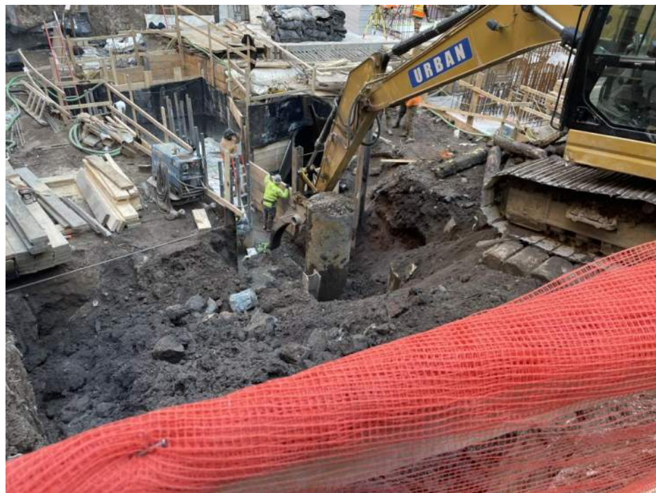
Photo 2: Urban excavating soil/fill in grid WC02 (facing northeast).
