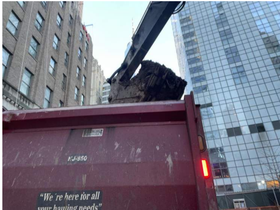
Photo 1: Urban loading a truck for soil/fill export (facing south).
