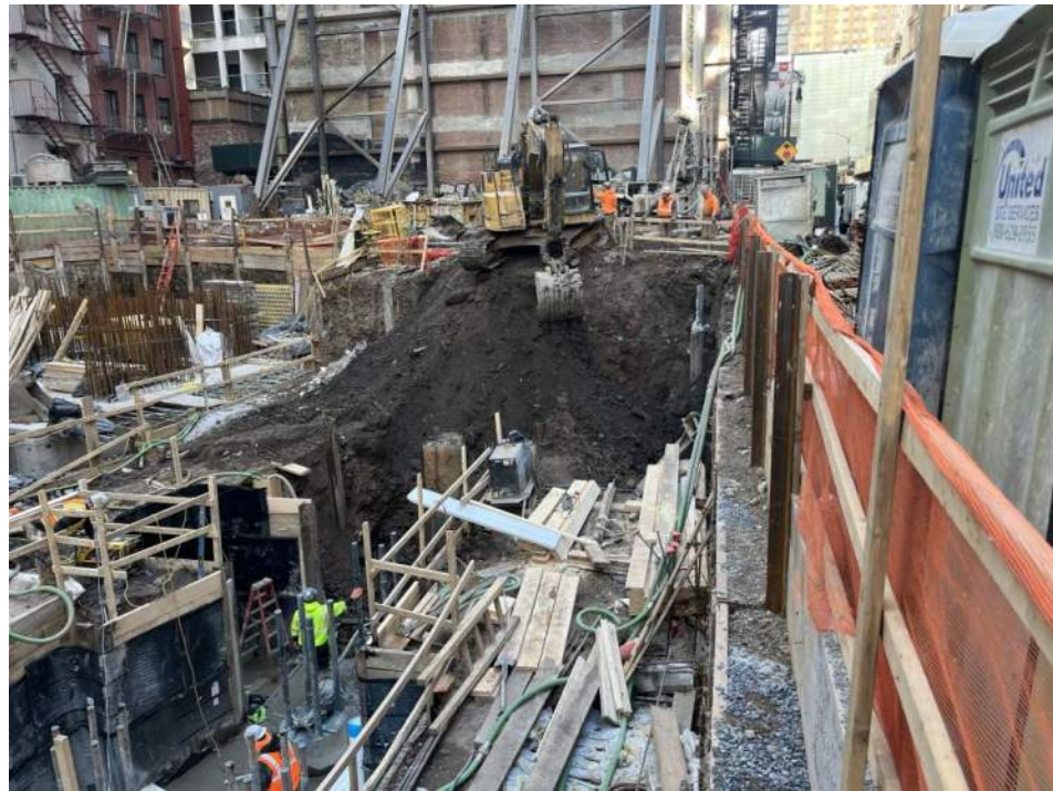
Photo 2: Urban grading soil/fill in grid WC02 (facing south).
