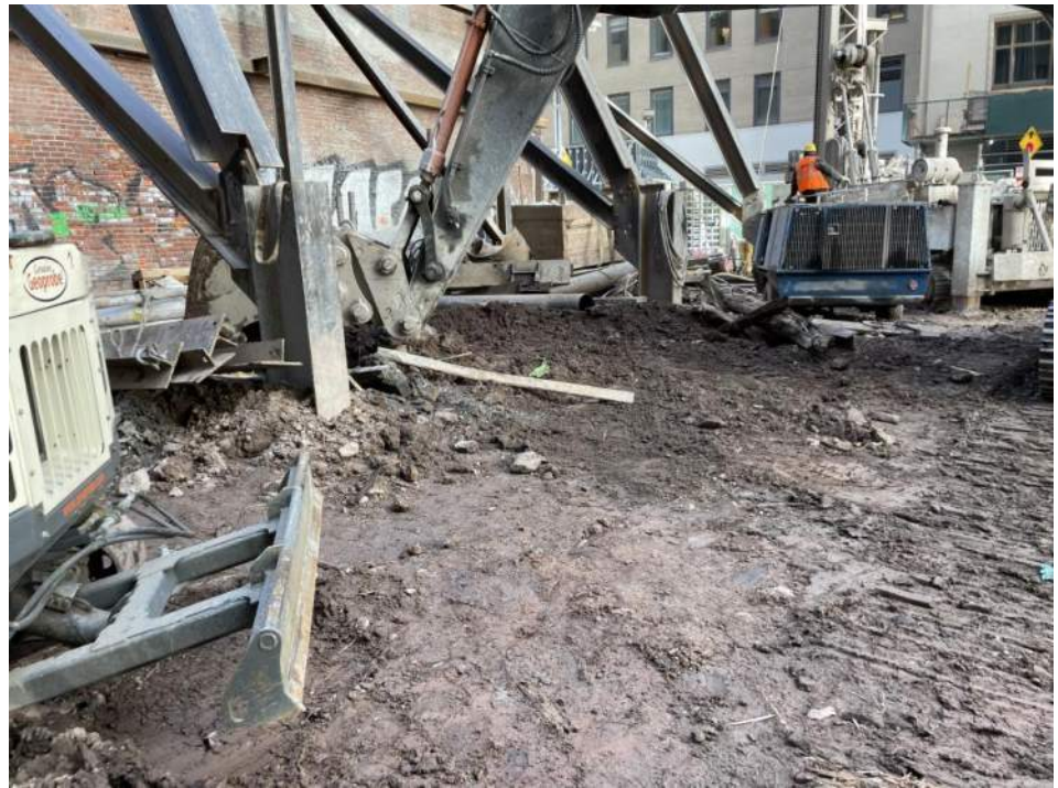
Photo 2: Urban excavating soil/fill in grid WC05 (facing southwest).
