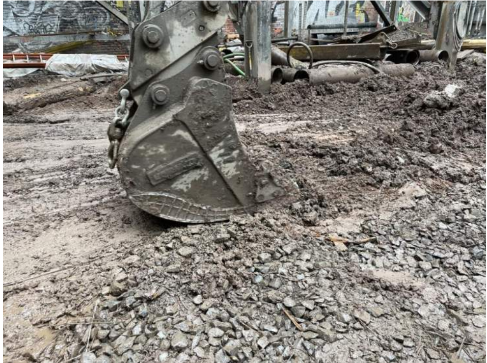
Photo 1: Urban grading soil/fill in WC05_0-5 (facing southwest).
