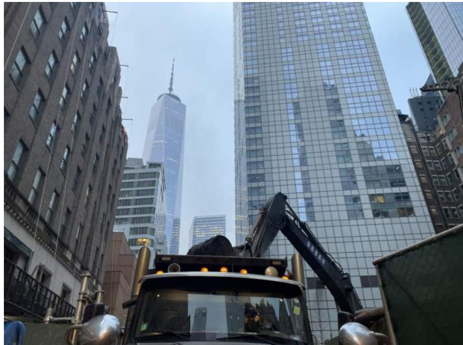
Photo 2: Urban loading a truck for soil/fill export (facing south).
