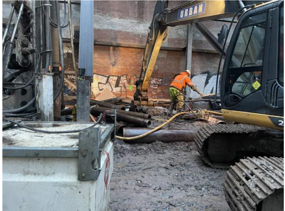
Photo 1: Urban excavating in WC04_0-5 (facing southwest).
