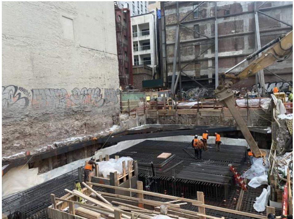
Photo 2: General view of the site (facing southeast).
