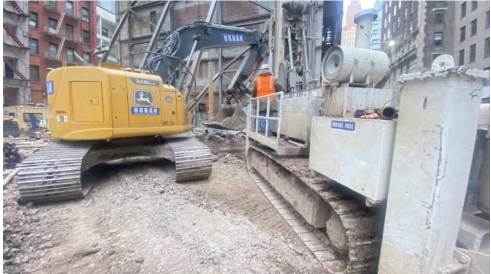
Photo 1: Urban grading in the western part of grid WC04 (facing southeast).
