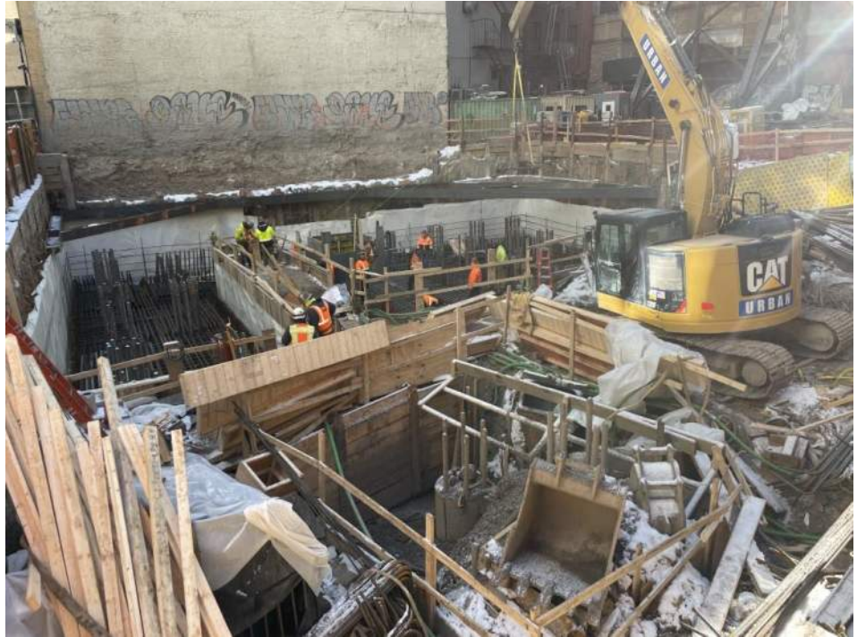
Photo 1: View of the eastern portion of the site (facing southeast).
