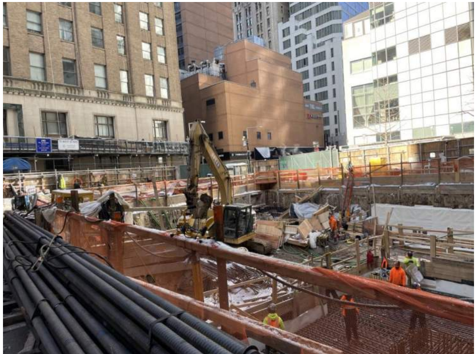
Photo 2: Urban reconsolidating and grading soil/fill in WC02 (facing northeast).
