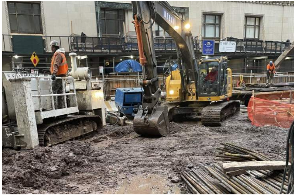
Photo 1: Urban grading soil/fill in grid WC04 (facing northwest).
