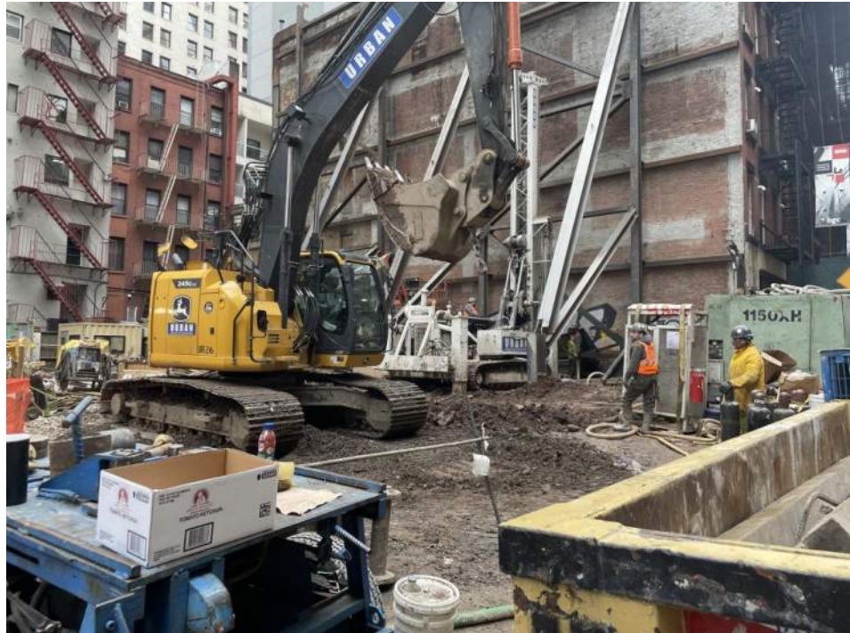
Photo 2: General view of the southern part of the site (facing southeast).
