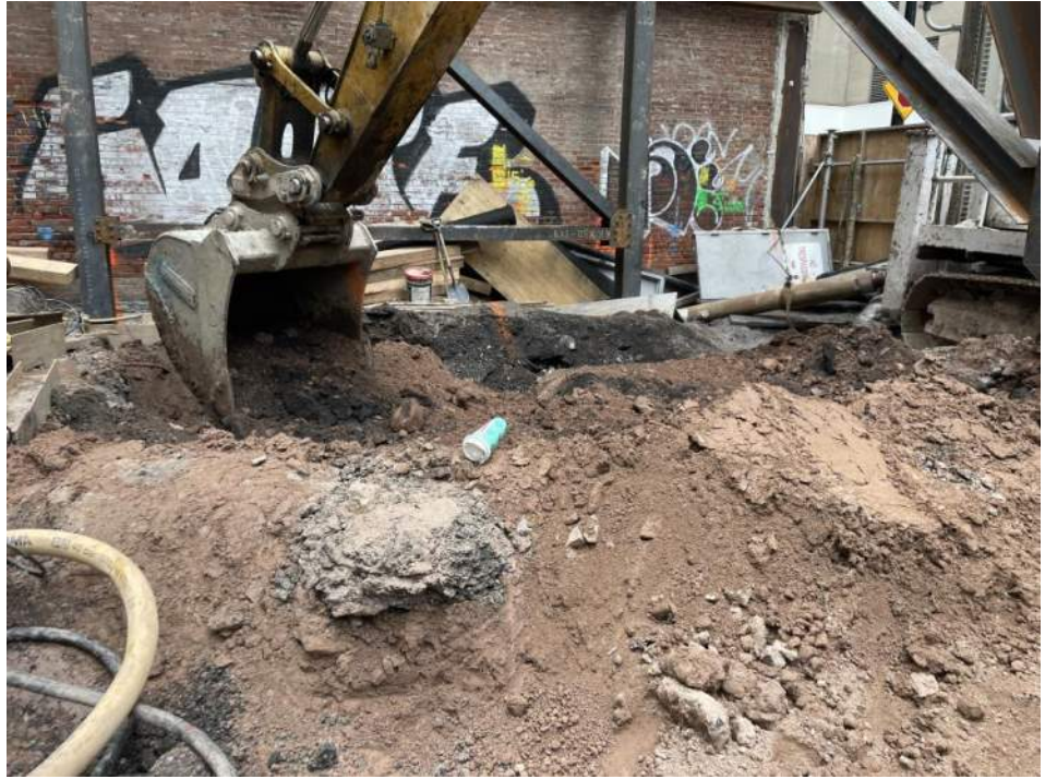
Photo 1: Urban excavating in the southern part of WC04_0-5 (facing southwest).
