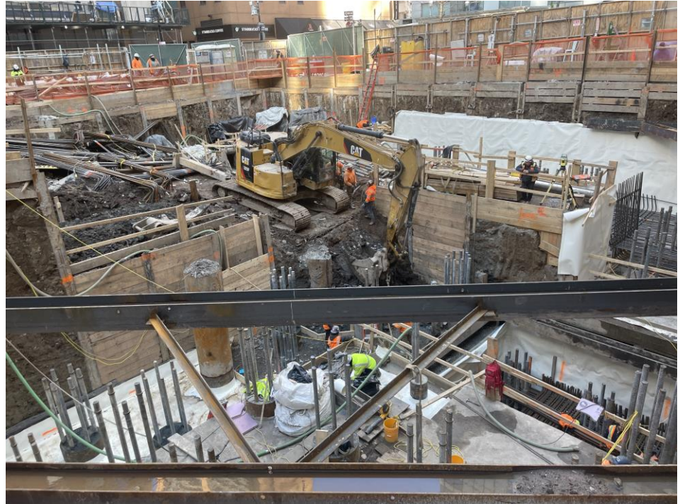
Photo 1: Urban excavating in the south-central part of WC03_15-20 (facing northwest).
