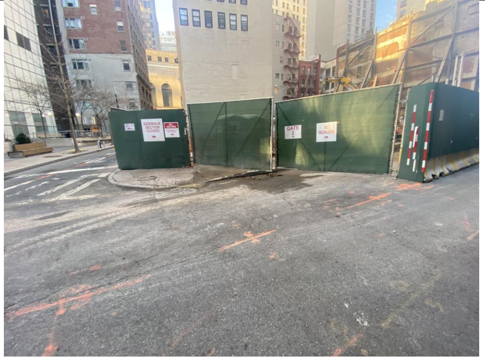
Photo 3: View of the site entrance/exit on the corner of Carlisle Street and Washington Street at the end of the workday (facing southeast).
