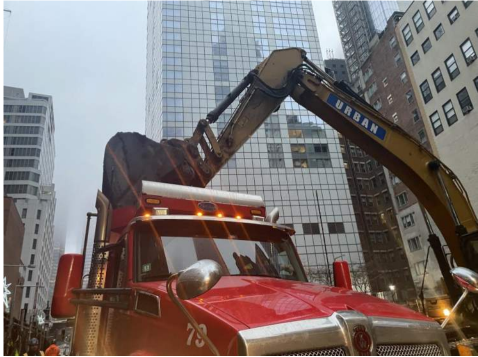
Photo 1: View of Urban loading a truck with soil/fill for off-site disposal (facing northeast).
