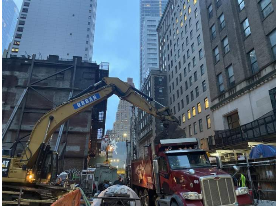
Photo 1: View of Urban loading a truck with soil/fill for off-site disposal (facing southwest).
