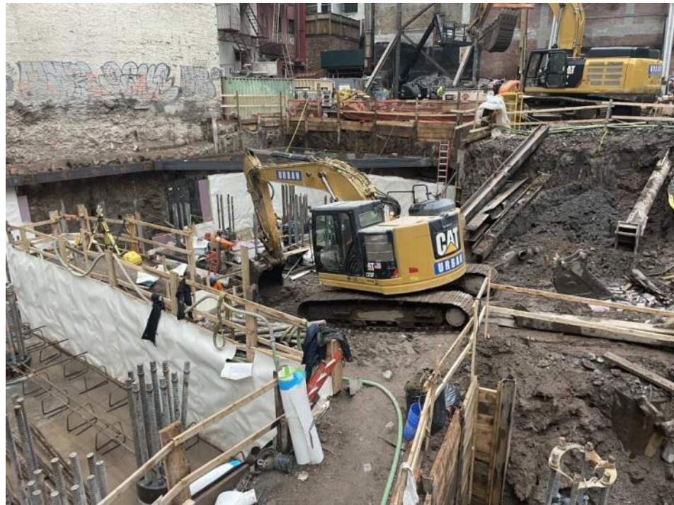
Photo 2: View of Urban excavating soil/fill in WC03_10-15 (facing southeast).
