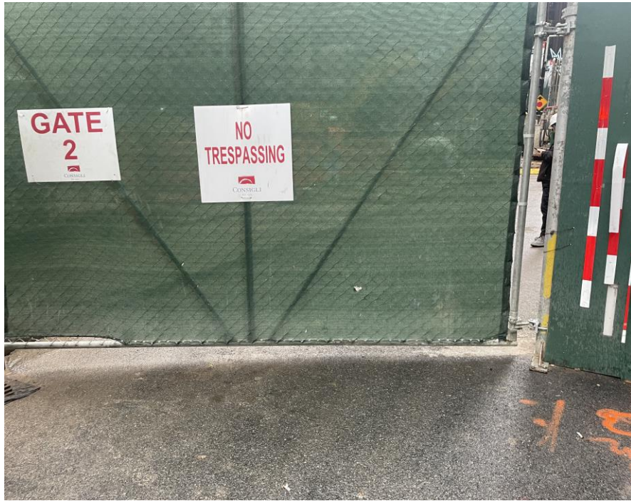
Photo 3: View of the site entrance/exit on the corner of Carlisle Street and Washington Street at the end of the workday (facing southeast).
