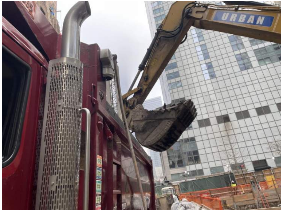
Photo 1: View of Urban loading a truck with soil/fill for off-site disposal (facing north).
