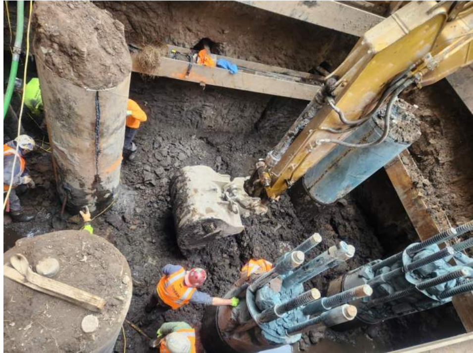
Photo 1: View of Urban excavating soil/fill in grid WC06_30-35 (facing southwest).
