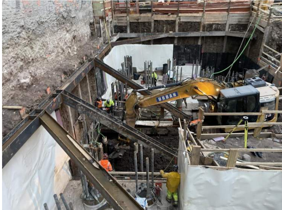
Photo 1: View of Urban excavating soil/fill in grid WC06_30-35 (facing south).
