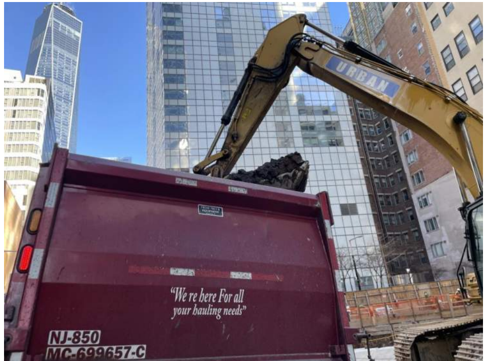
Photo 2: View of Urban loading a truck with soil/fill for off-site disposal (facing northeast).
