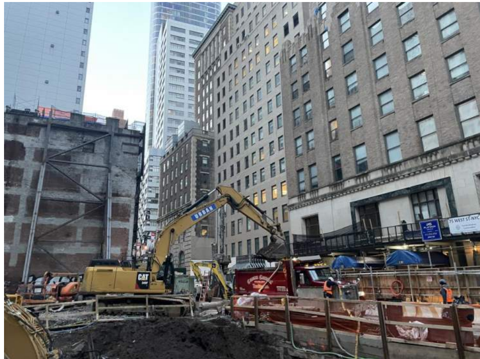
Photo 2: View of Urban loading a truck with soil/fill for off-site disposal (facing southwest).
