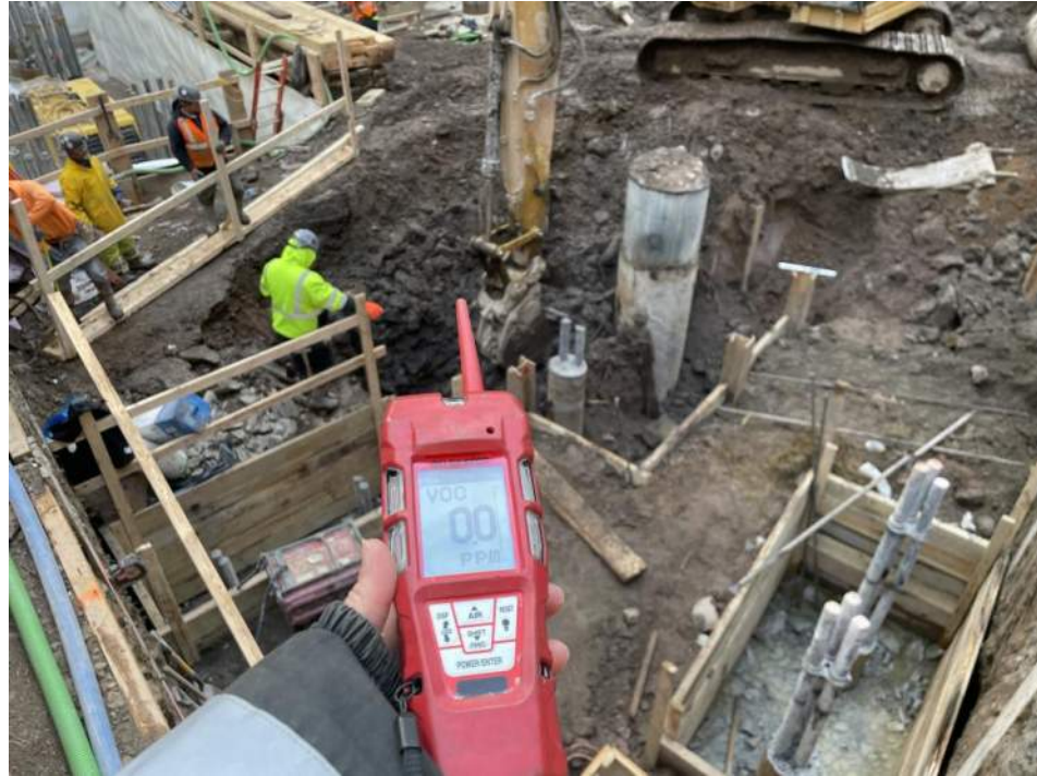
Photo 1: View of Urban excavating soil/fill in WC02_15-20 (facing southeast).
