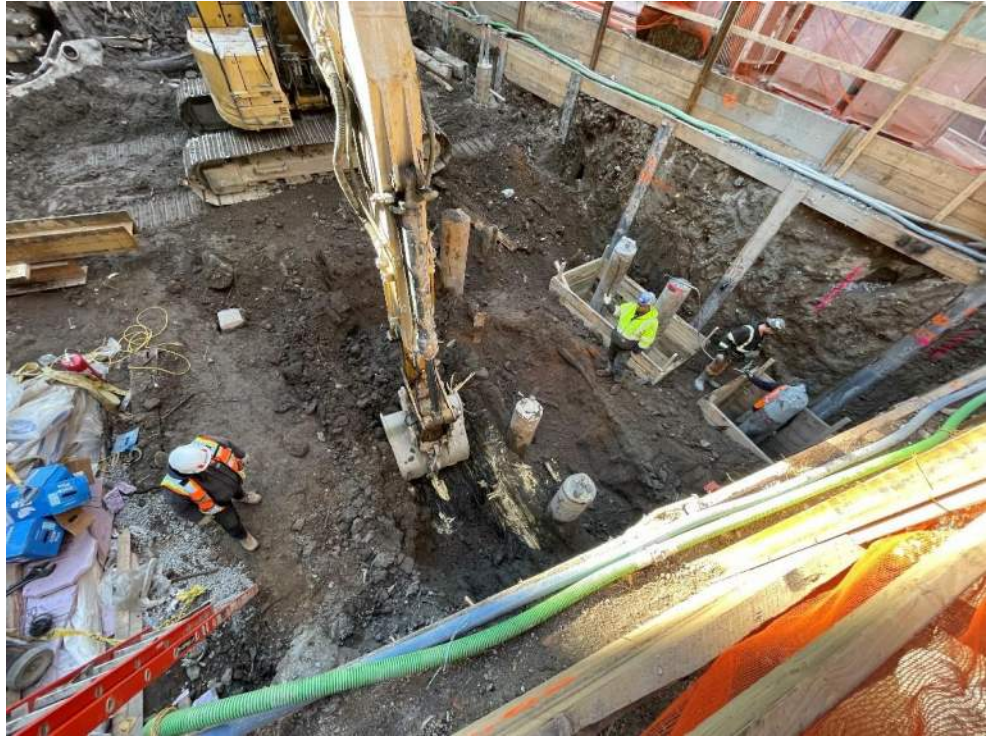
Photo 1: View of Urban excavating soil/fill in WC02_10-15 (facing southwest).
