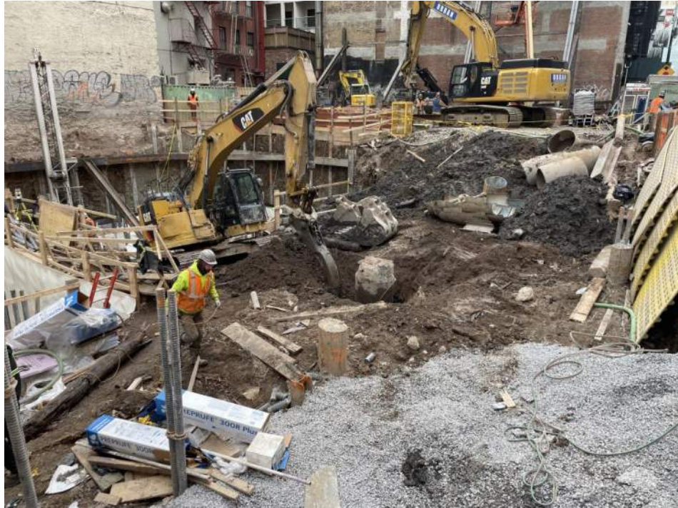
Photo 1: View of Urban excavating soil/fill in WC02_5-10 (facing southeast).
