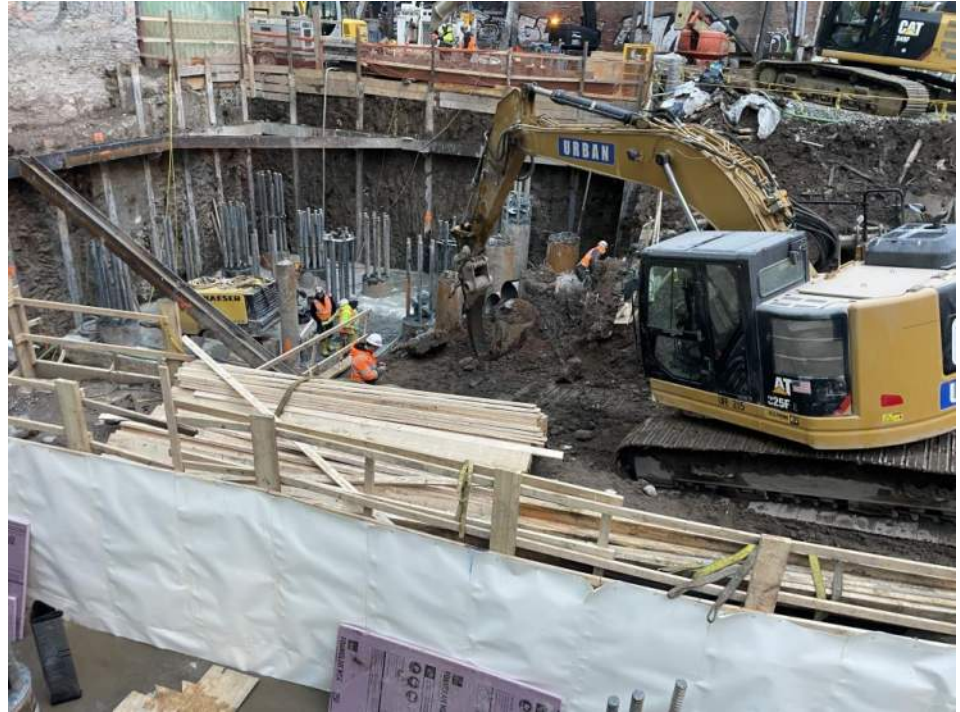
Photo 1: View of Urban excavating soil/fill in WC03_10-15 (facing southeast).
