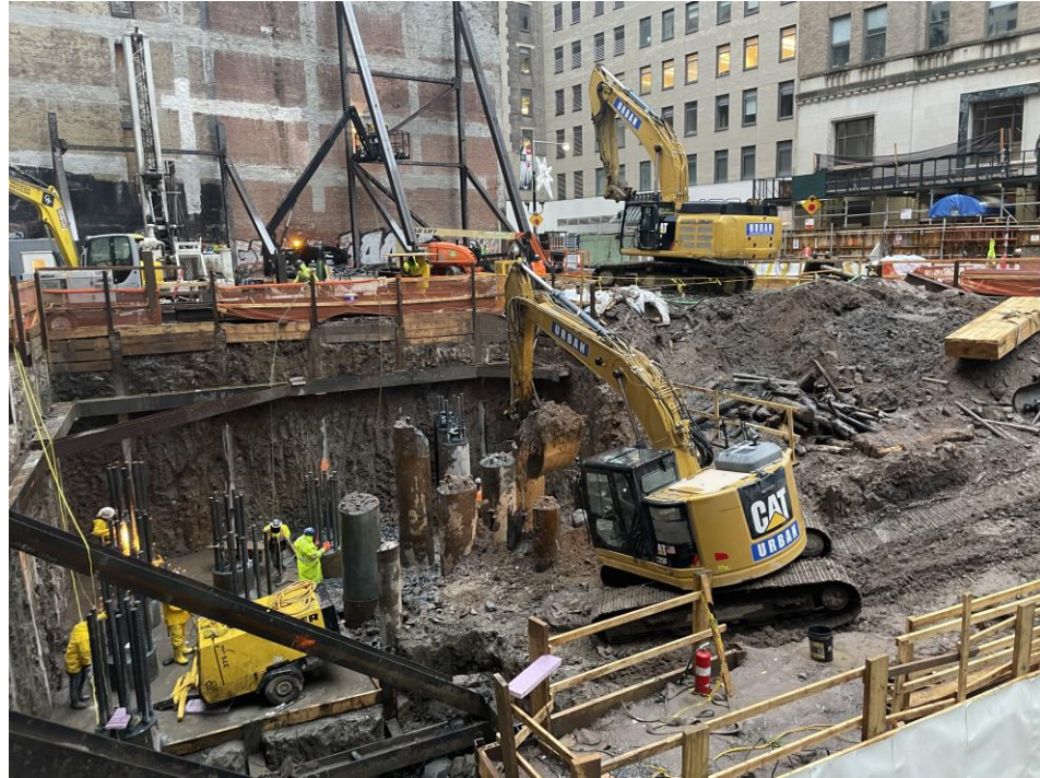
Photo 1: View of Urban excavating soil/fill in WC03_15-20 (facing southeast).
