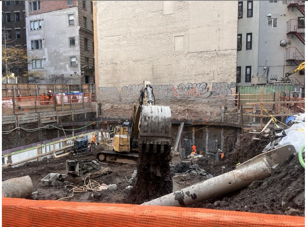
Photo 2: View of Urban stockpiling soil/fill in the western part of the site (facing east).
