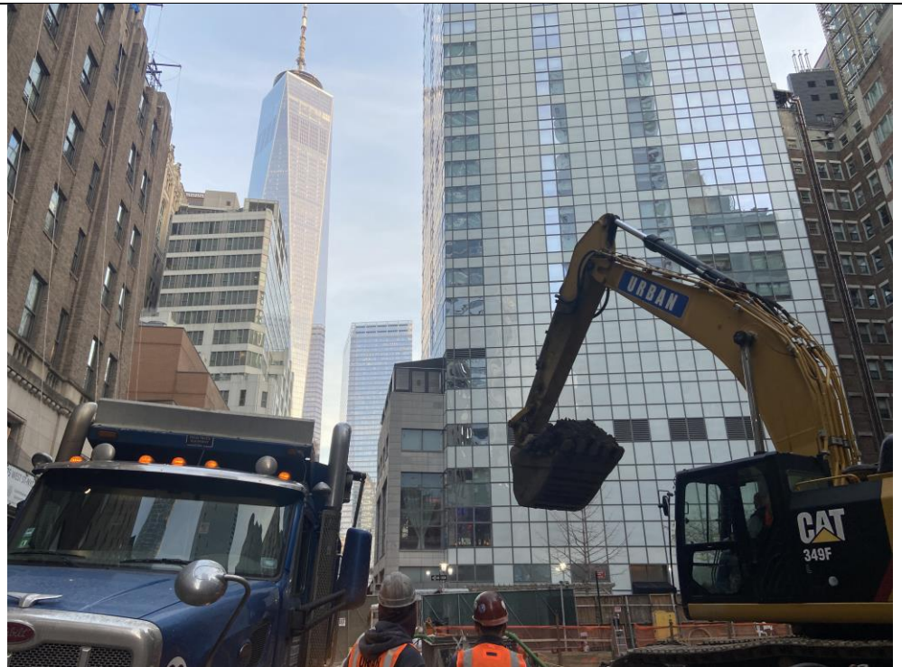
Photo 2: View of Urban loading soil/fill for (facing north).
