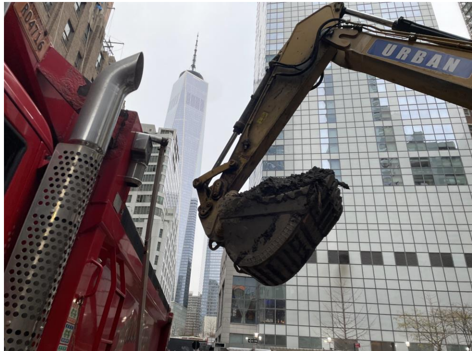
Photo 2: View of Urban loading soil/fill for (facing northeast).
