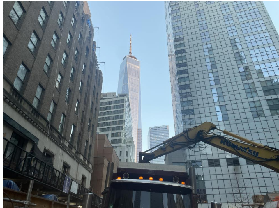
Photo 2: View of Urban loading soil/fill for (facing northwest).
