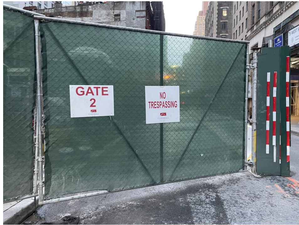
Photo 3: View of the site entrance/exit at the corner of Carlisle and Washington Street at the end of the workday (facing south).
