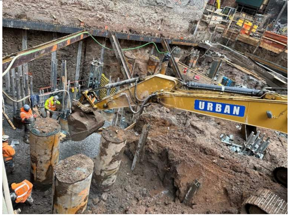
Photo 1: View of Urban backfilling 0.75-inch stone in grid WC03 (facing southeast).
