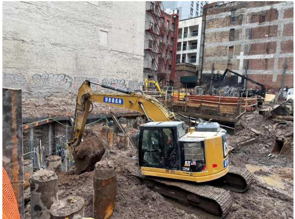
Photo 2: View of Urban excavating in grid WC03 (facing northeast).
