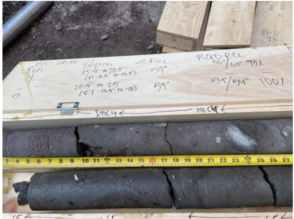
Photo 3: View of a collected soil mix core from the center of the ISS Columns.
