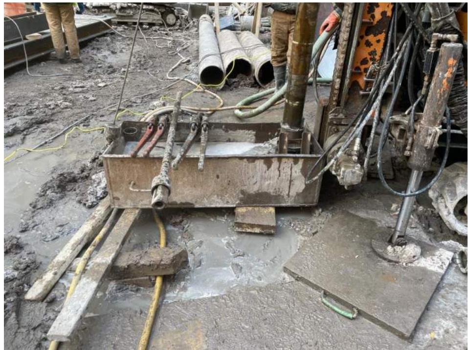
Photo 2: View of ADT advancing a core at ISS column #2B (facing east).
