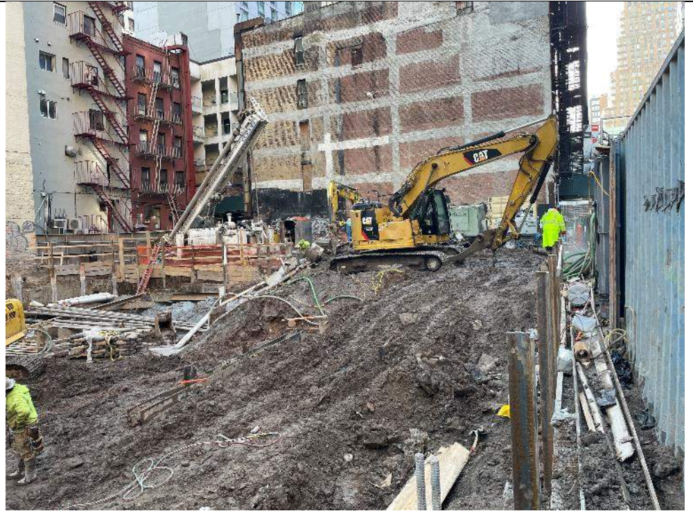
Photo 1: General view of the the site (facing southeast).
