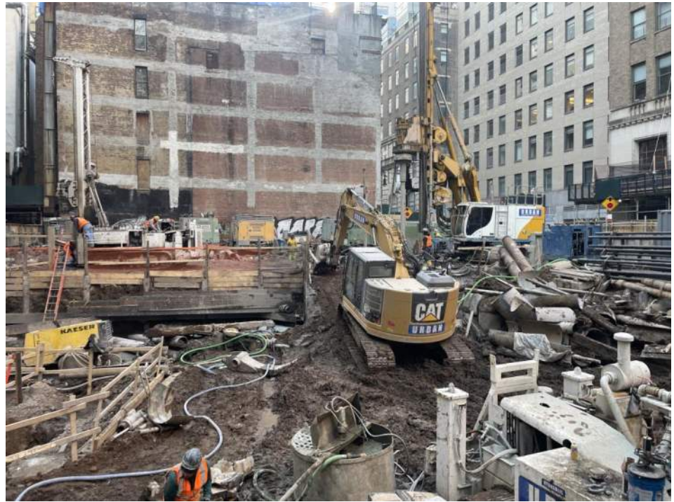
Photo 1: View of Urban excavating soil/fill in WC04 (facing southwest).
