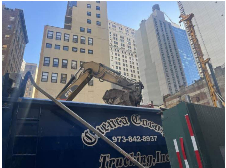
Photo 1: View of Urban loading a tri-axial truck with soil/fill for off-site disposal (facing east).
