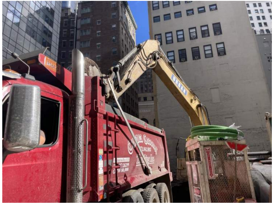
Photo 1: View of Urban loading a tri-axial truck with soil/fill for off-site disposal (facing northeast).
